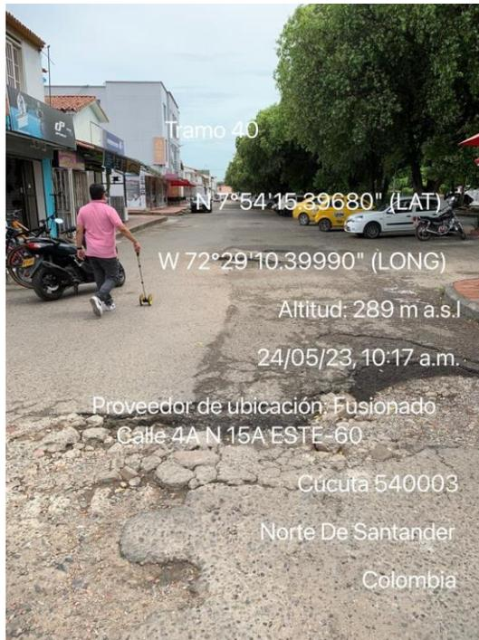
**SEGMENTO 40: ENCONTRAMOS UN TIPO DE PAVIEMNTO FLEXIBLE EN MAL ESTADO CON PIEL DE COCODRILO, HUNDIMIENTOS, BACHES.**
